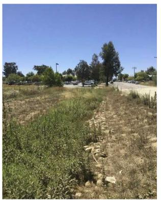
19. View of stormwater detention swale between 13th street road and Basin 1. This receives water from the paved 13th street to the south.
