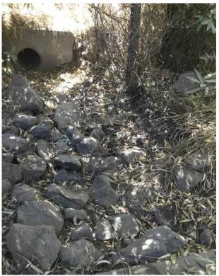
21. View of stormwater culvert and detention basin that drains Basin 1. This receives water from the library parking lot and the stormwater detention swale/13th street.
