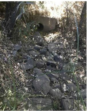
24. View of stormwater culvert and basin that drains Basin 1. This receives water from the library parking lot and the stormwater detention swale/13th street.
