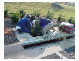
• After removal of mulch and debris, measure distance from the top of the Filterra engineered media soil to the top of the top slab. Compare the measured distance to the distance shown on the approved Contract Drawings for the system. Add Filterra media (not top soil or other) to bring media up as needed to distance indicated on drawings.
