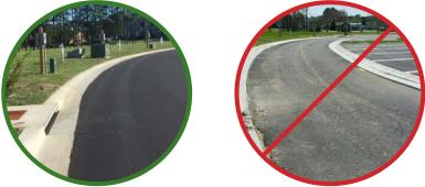
3. Filterra throat opening should be at least 4" in order to ensure adequate capacity for inflow and debris.
