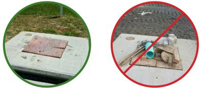
2. Final paving must be completed. Final paving ensures that paving materials will not enter and contaminate the Filterra system during the paving process, and that the plant will receive runoff from the drainage area, assisting with plant survival for the Filterra system.
