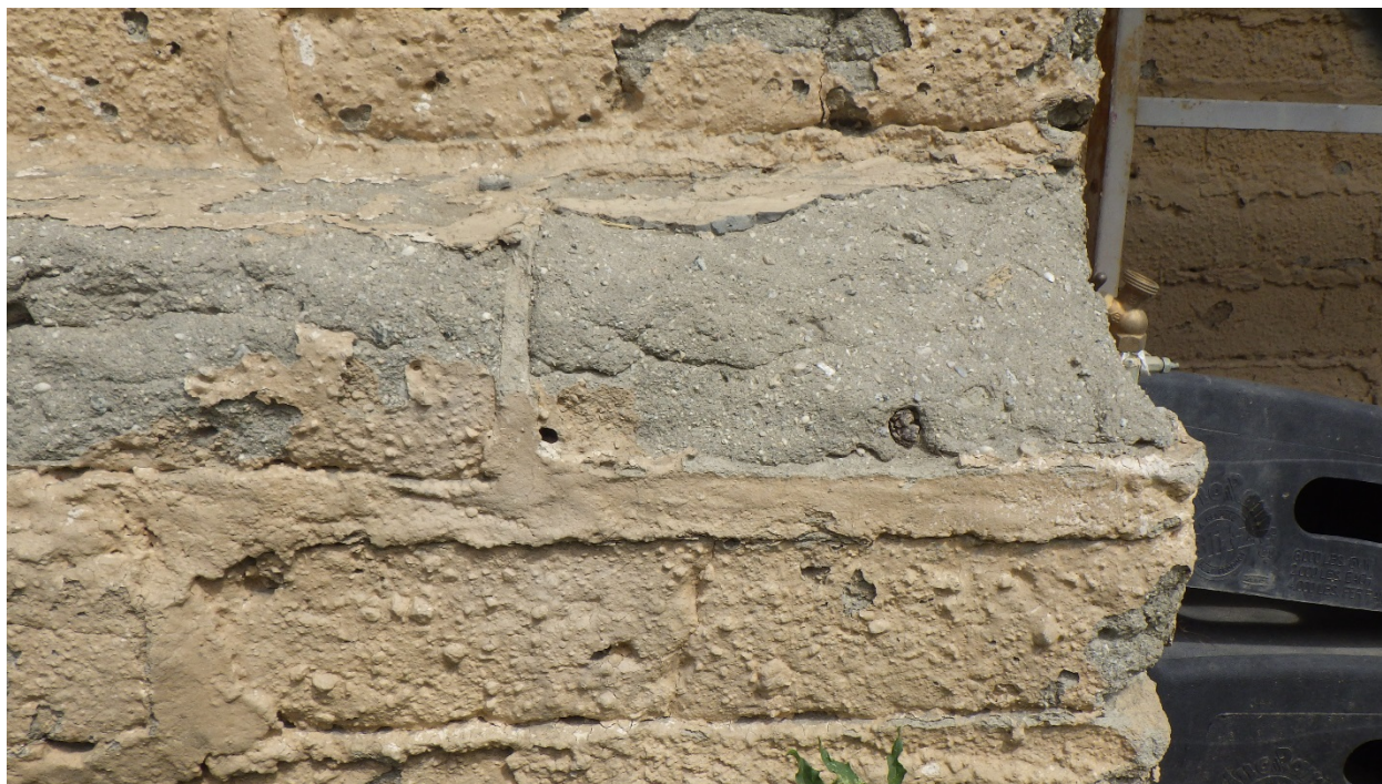
Photograph 6-10. Adobe brick with paint covering.
