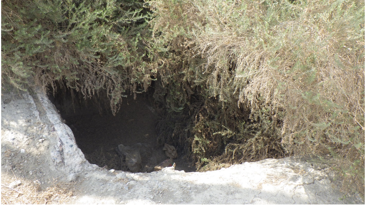
Photograph 6-16. Section of levee nearest to 66 th Ave, showing degradation and vegetation
