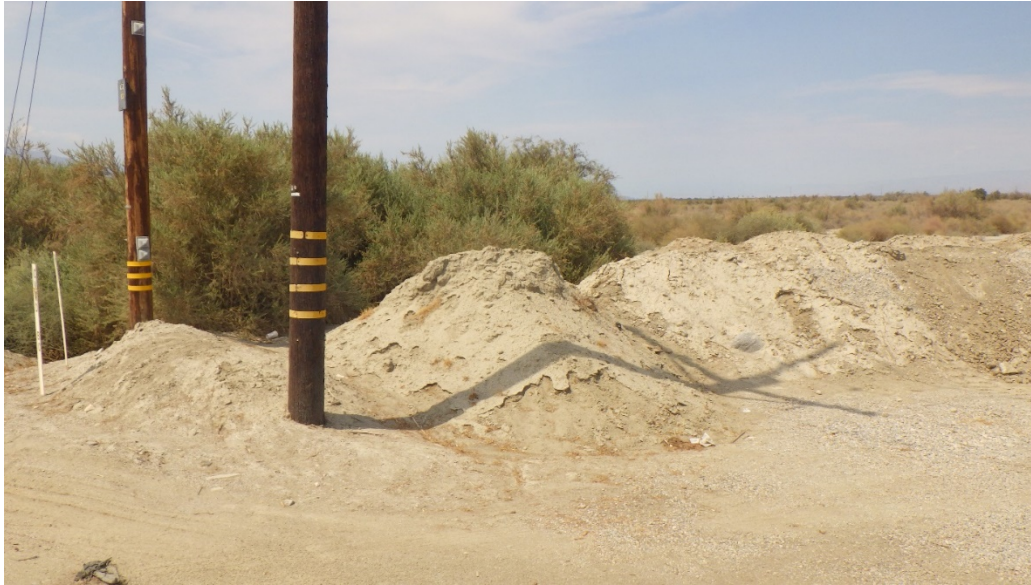
Photograph 5-8. Heavy vegetation growing inside of and around the levee
