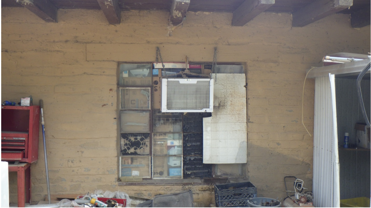
Photograph 6-13. Boarded window with brick sill
