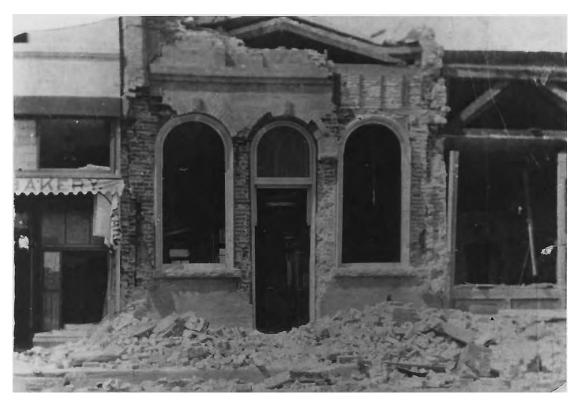
Figure 10: Photograph of the damage to the Bank of Sebastopol (no longer extant) on Main Street near Bodega Avenue caused by the 1906 earthquake (Courtesy of the Sonoma County Library).
