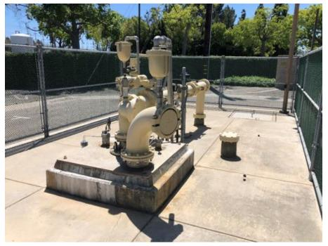
Figure 4-5. Example Injection Well Site
