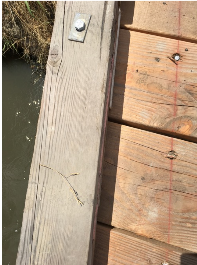
Photo 9 – Wooden decking and curb rail.
