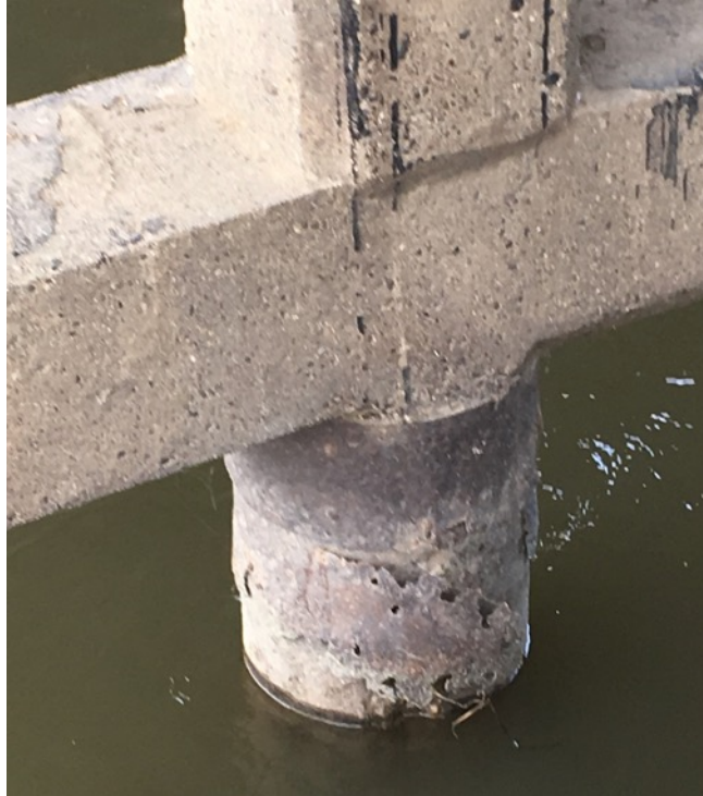
Photo 5 – Corroded steel jacketing on pile (western pier).
