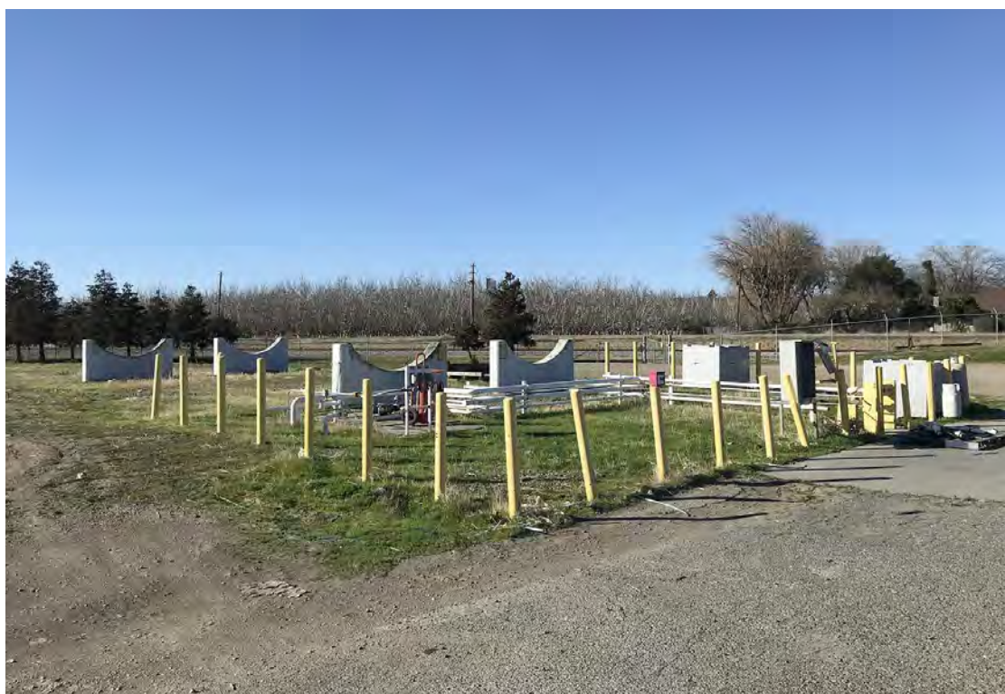
Photo No. 54 View to the southwest of former propane AST saddles west of the north warehouse
