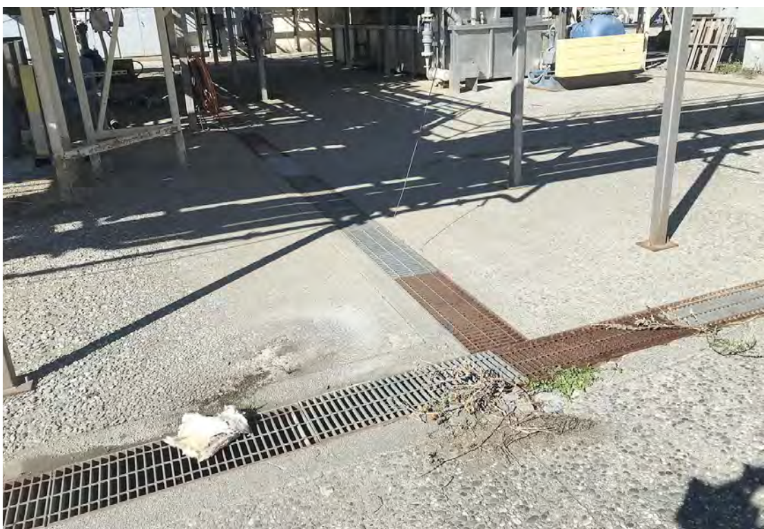
Photo No. 24 Trench drains beneath the peeler area
