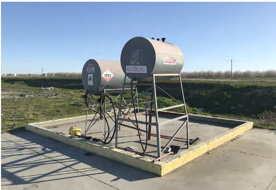
Photo No. 61 Diesel (left) and gasoline (right) ASTs southwest of the emergency wastewater discharge pond
