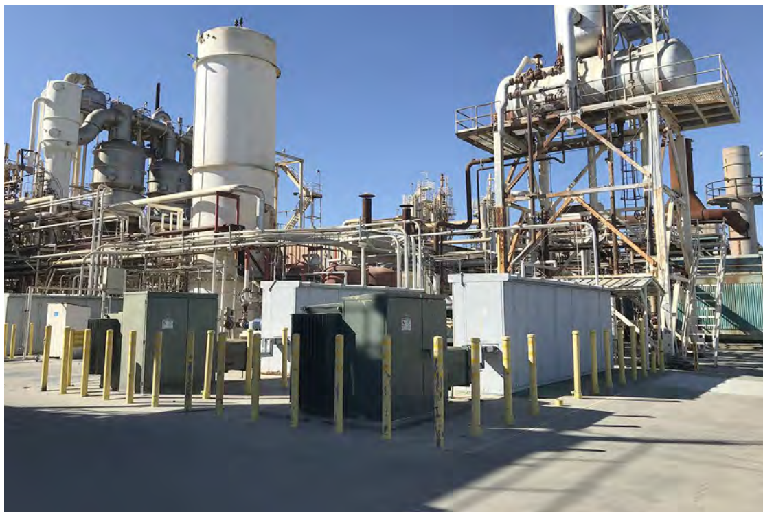
Photo No. 28 View to the southwest of water softener equipment north of the boiler room and water tanks with associated piping, pad-mounted transformers, and electrical cabinets east of the boiler room
