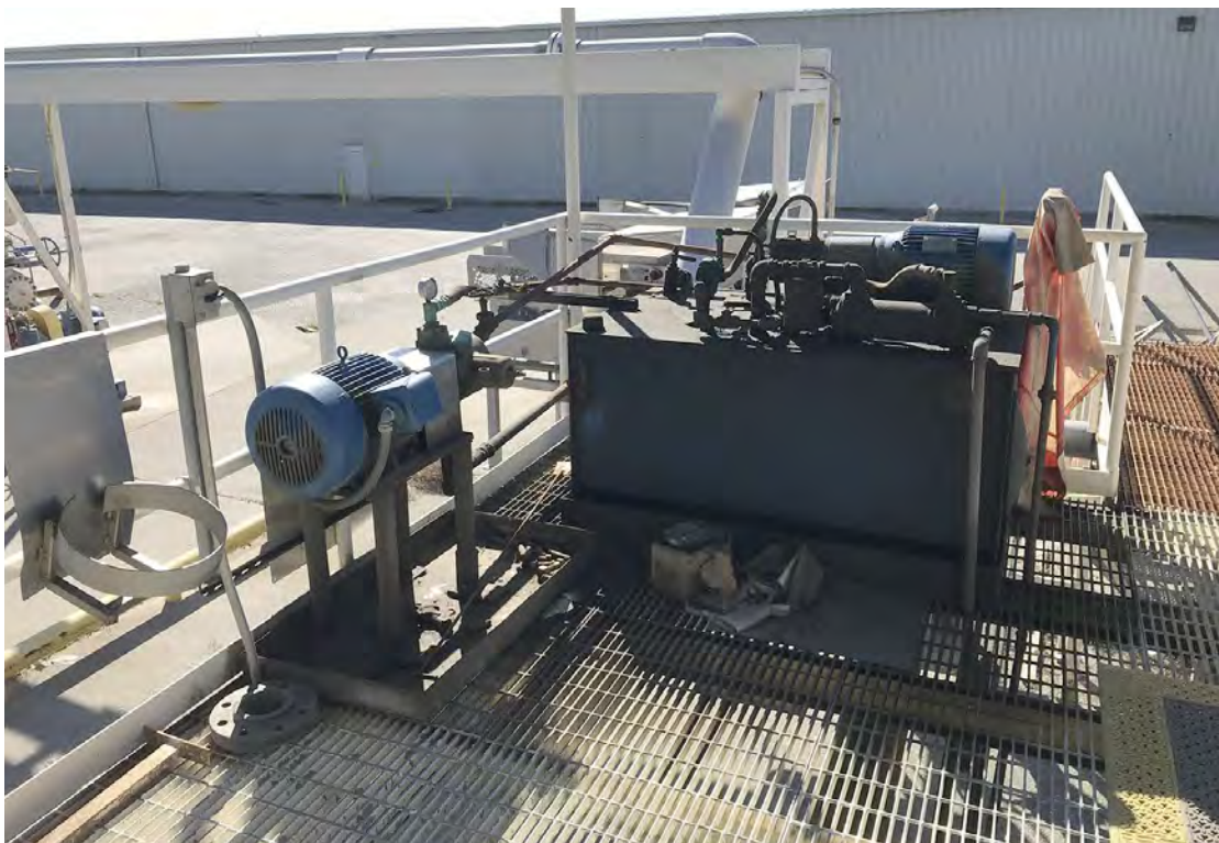
Photo No. 25 Hydraulic fluid tank and equipment in the bulk tomato dump area
