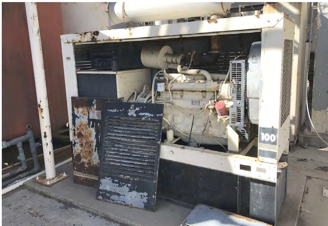
Photo No. 29 Diesel-powered generator east of the boiler room
