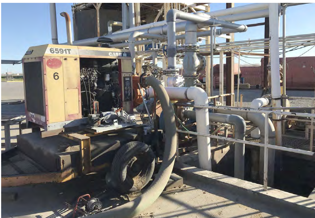
Photo No. 62 Diesel-powered backup power generator and separator at the pump station
