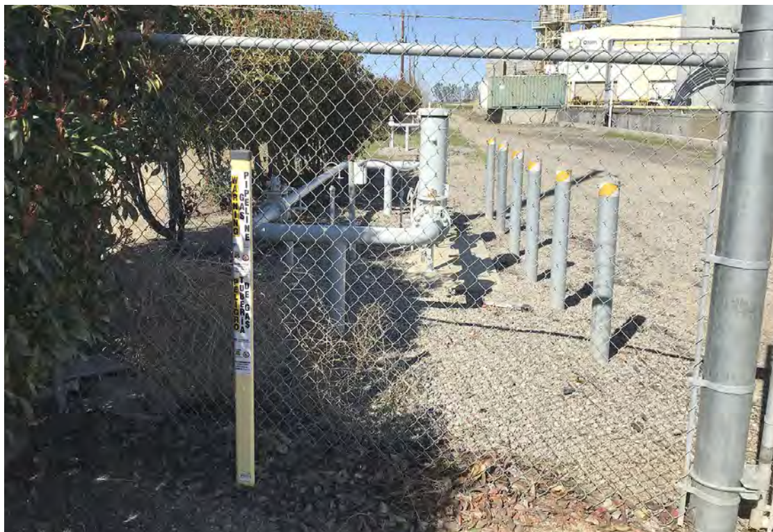
Photo No. 9 Marker in southwestern portion of the Site indicating a buried natural gas pipeline along the western site boundary
