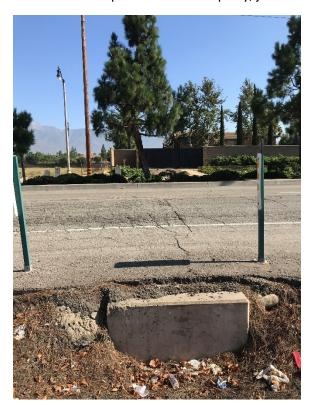
Photo 16 – Concrete block abutting East Foothill Boulevard at northern end of the earthen swale. This location appeared to be an area where stormwater historically was conducted beneath the road and onto the Property.
