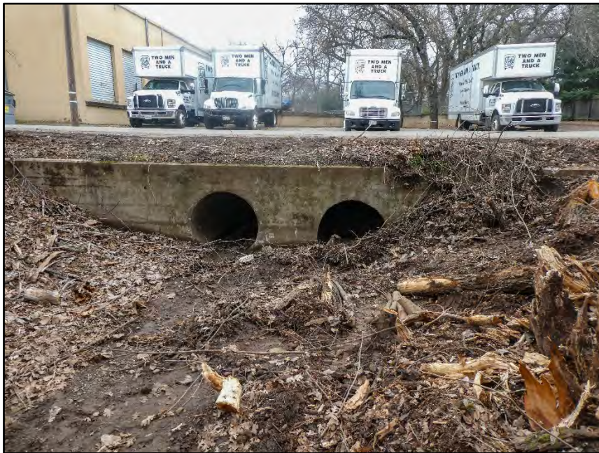
Water enters the swale through two culverts underneath Comanche Court at the study area's eastern boundary. Photo Date 01-20-20.
