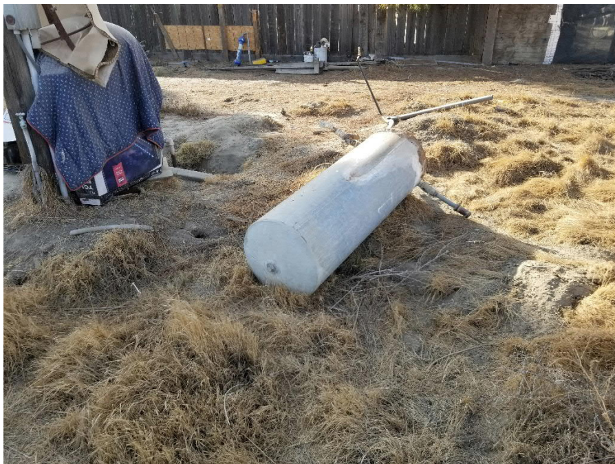
Photo 48: View of domestic well and previous pressure tank near the eastern boundary of the furthest residence west on South 19th Avenue. Although not a REC any well which is not going to remain in use should be properly abandoned in accordance with state and local regulations.
