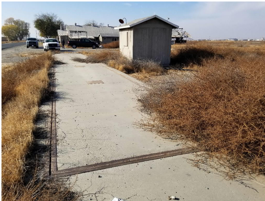
Photo 2: View of scale and associated structure adjacent to abandoned dairy building. It is unknown if it is mechanical or hydraulic. Scales have the potential to leak hydraulic fluid without observation. This scale qualifies as a REC.
