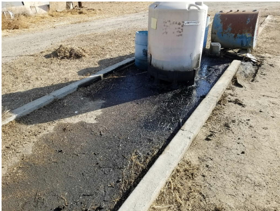
Photo 38: View of ASTs, 55-gallon drums, spillage, and surface staining east of livestock building. Concrete and soil staining appears to be related to petroleum products. This release qualifies as a REC.
