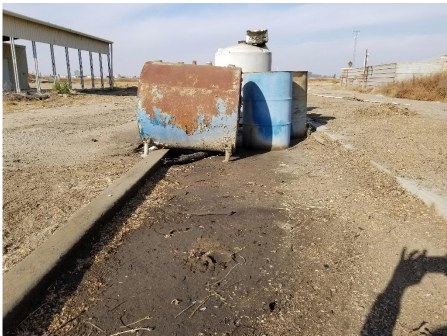
Photo 40: View of staining and spillage area from the south. Concrete and soil staining appears to be related to petroleum products. This release qualifies as a REC.
