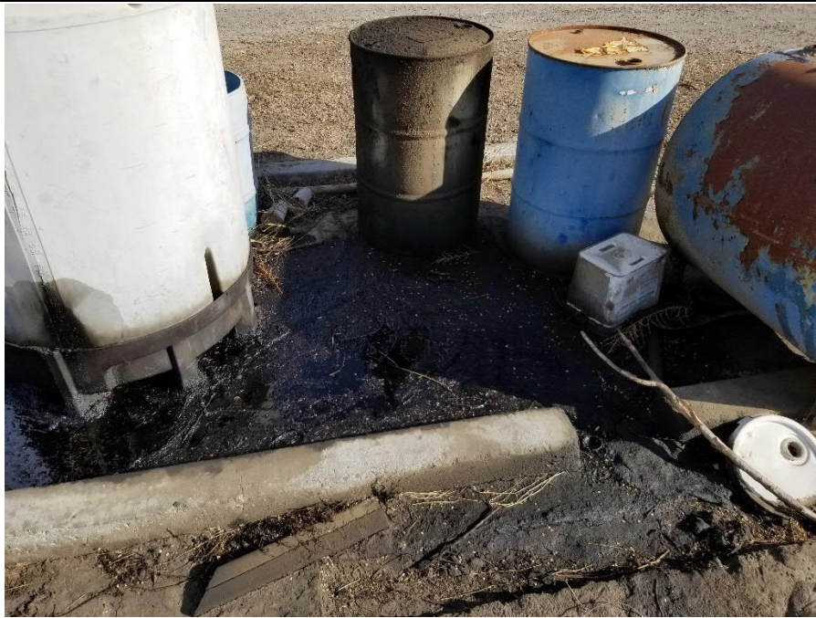
Photo 39: View of spillage and staining area showing extent and a break in the in the concrete allowing hazardous materials to impact the soil. Concrete and soil staining appears to be related to petroleum products. This release qualifies as a REC.
