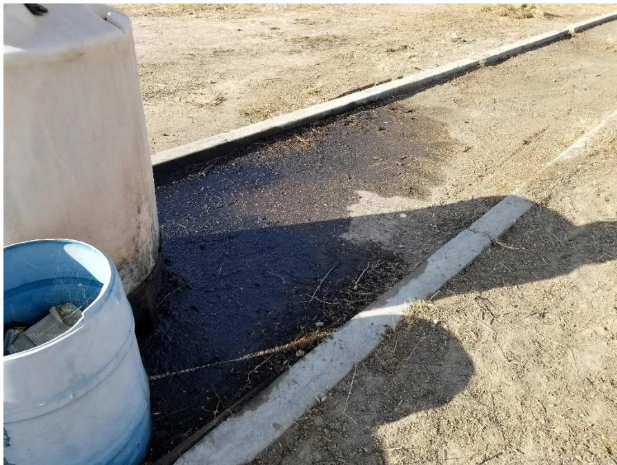
Photo 42: View of staining and spillage area form the east. Concrete and soil staining appears to be related to petroleum products. This release qualifies as a REC.
