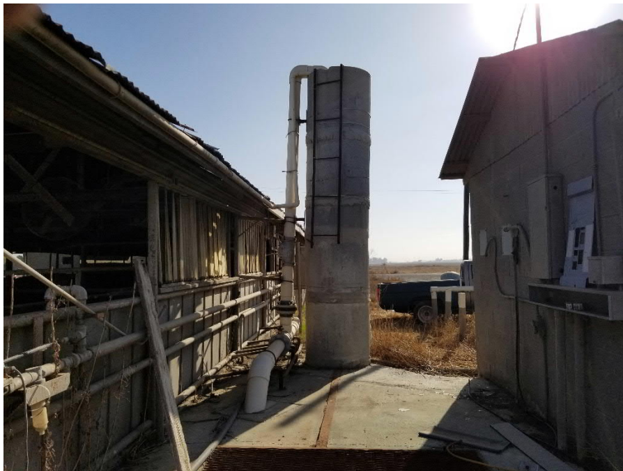
Photo 10: View of standpipe along western boundary of abandoned dairy building that empties into below grade vault. Use is believed to be either irrigational or part of stormwater collection system. The below grade vault has the potential to concentrate contaminants if used for stormwater or wastewater. This vault qualifies as a REC.
