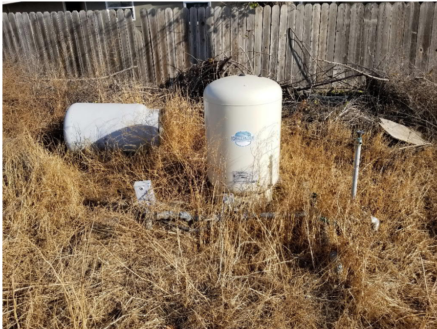
Photo 18: View of second well along western boundary of residence west of the abandoned dairy building. Although not a REC, any well that is not going to remain in use, should be abandoned in accordance with state and local regulations.
