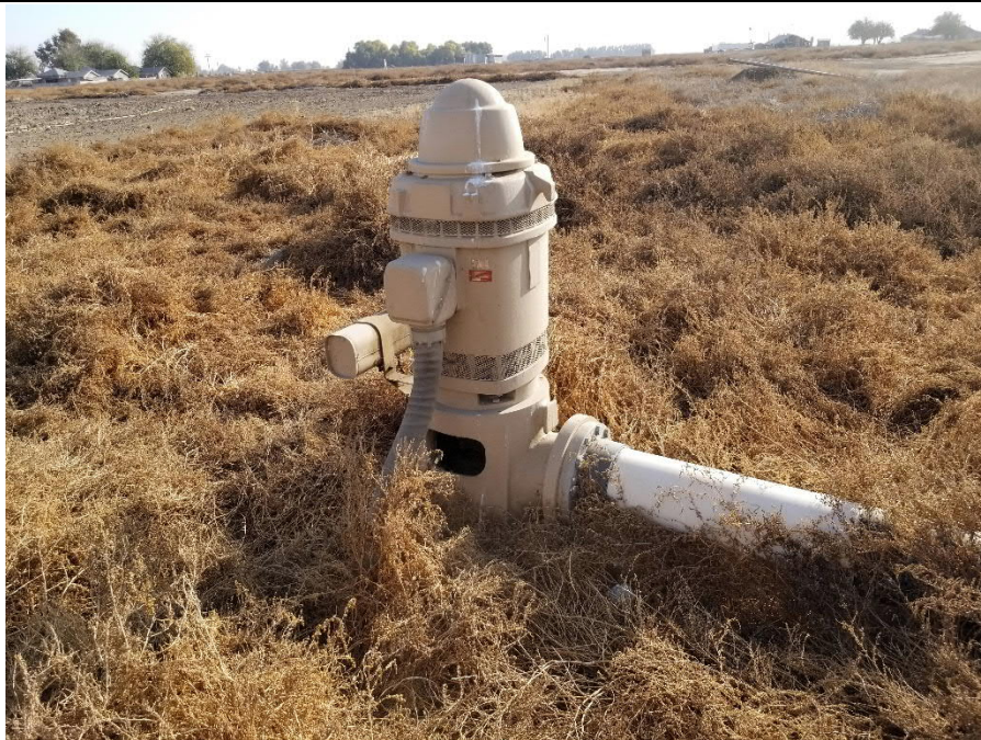
Photo 53: View of irrigation well with a vertical turbine pump located near southeast corner of the easternmost ponding basin (#4). Turbine-pumps can be either water or oil lubricated which can lead to unintended releases of oil into groundwater. Therefore, the potential release from this pump qualifies as a REC.
