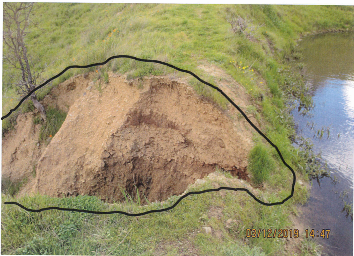
Attachment #2 Fill area black highlighted up to 250 cubic yards dam, use top soil from spill to revegetate dam face, Blue line is approx. location of 2 ft deep 5ft. wide 40 ft long dam base key per Geocon report.
