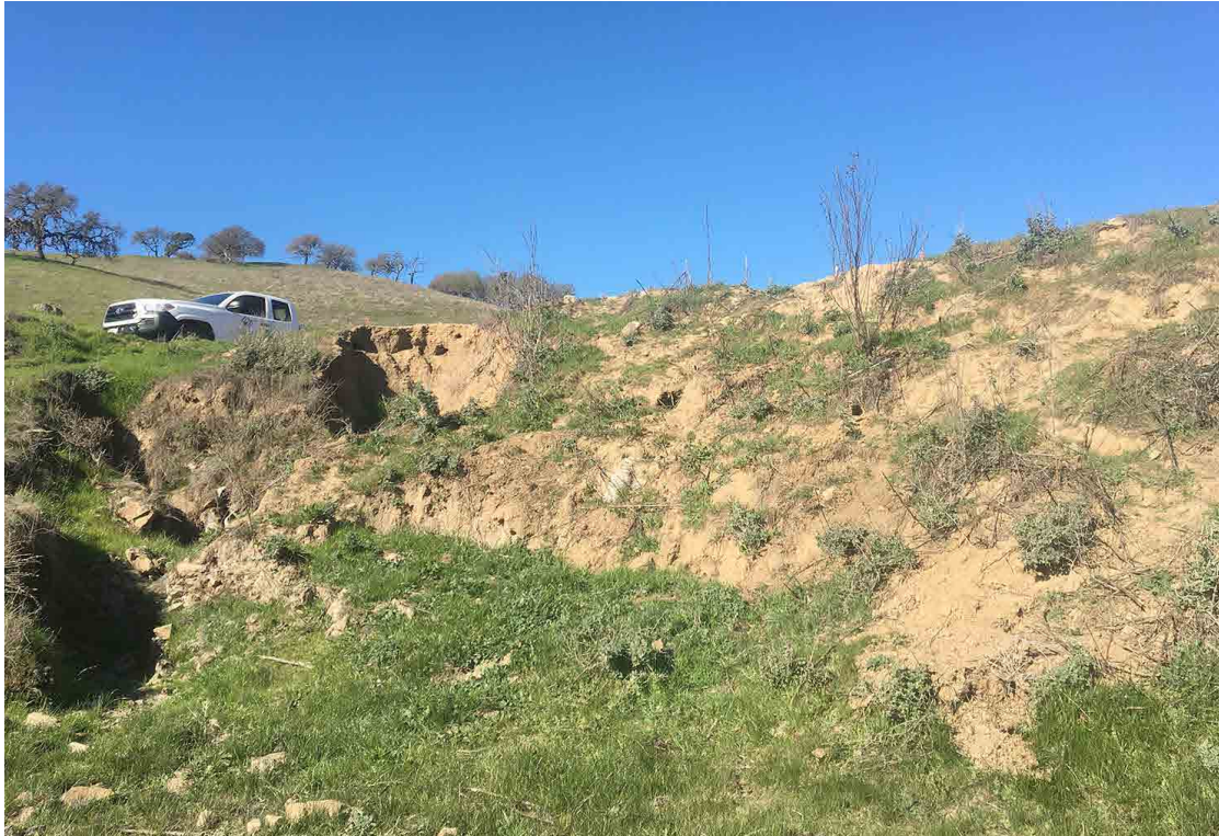
Photo No. 3 Pig Pond Dam looking north showing animal burrows in the dry side of the dam
