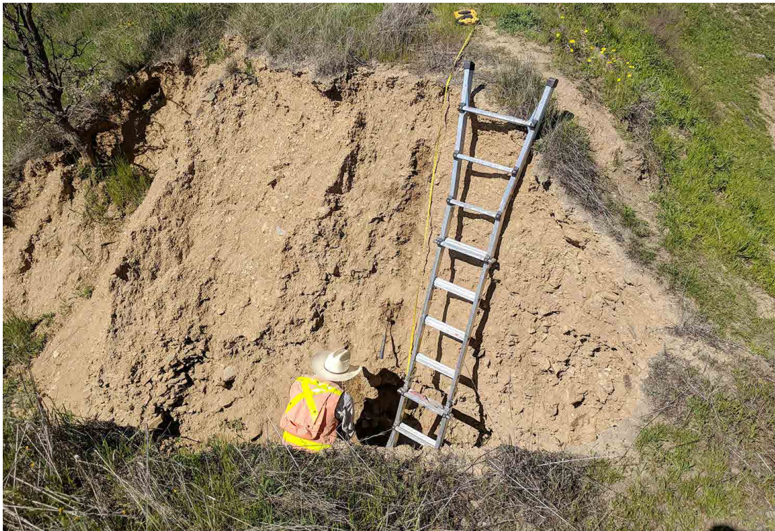
Photo No. 8 Bear Hide Lake Dam showing dam breach erosion
