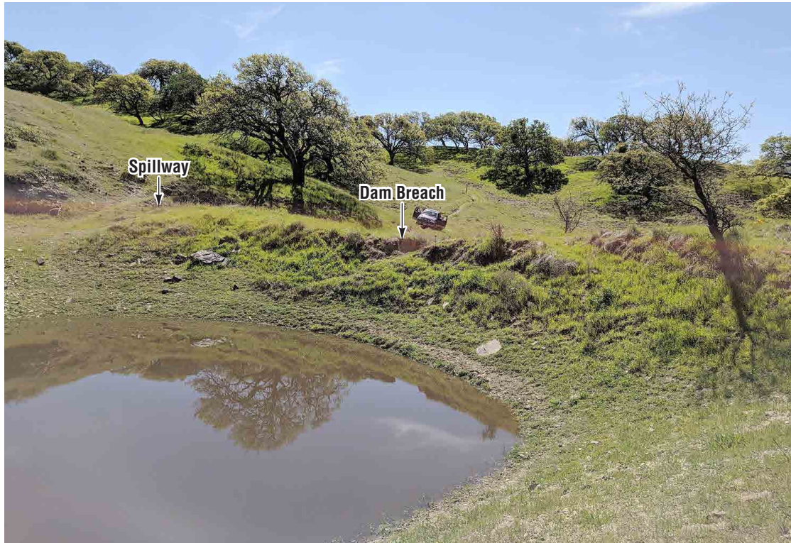
Photo No. 7 Bear Hide Lake Dam showing dam breach and spillway
