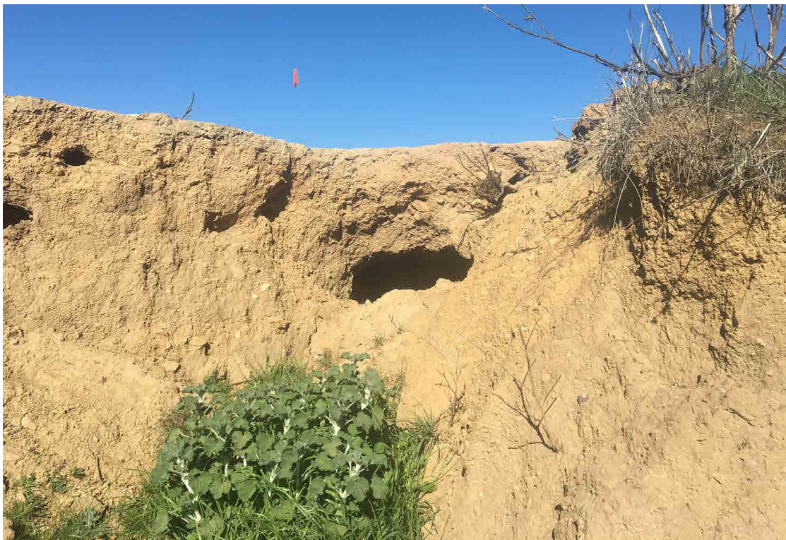
Photo No. 4 Animal burrows in the dry side of the dam
