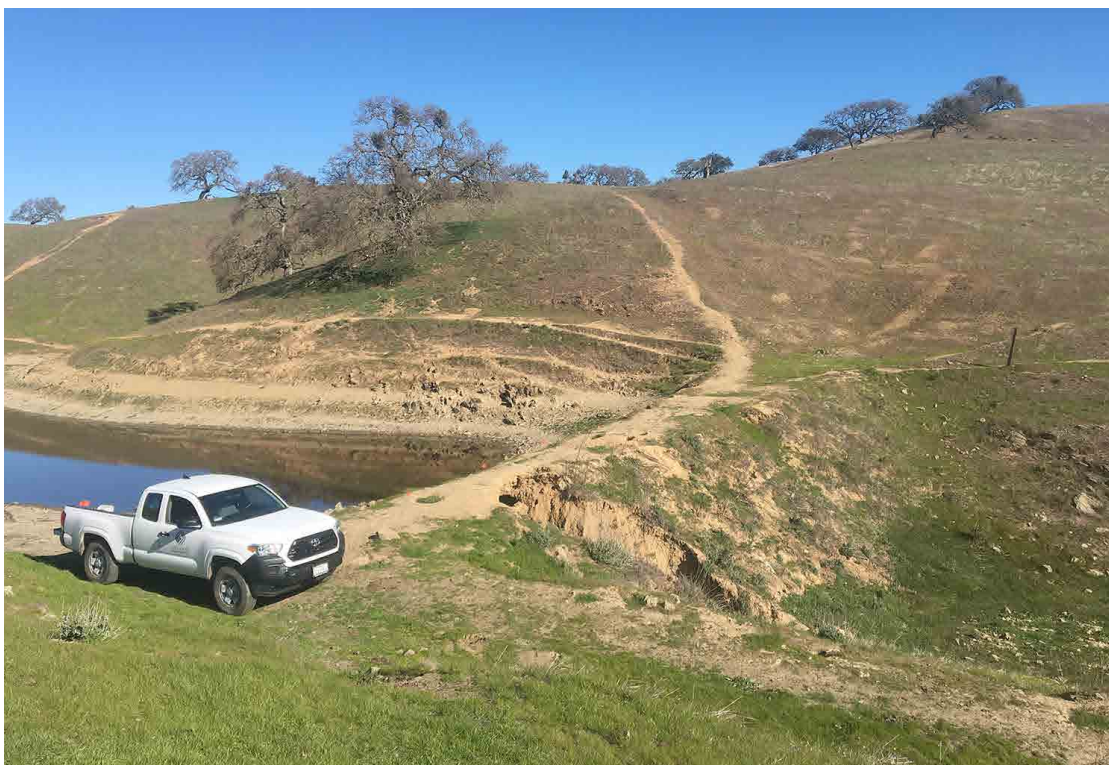
Photo No. 2 Pig Pond Dam looking east showing dam breach erosion in the foreground
