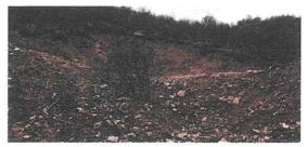
The damaged Lower Access Road is located on PG&E right of way, though UPRR accesses Tunnel Number 7 and Tunnel Number 8 from the Lower Access Road. This Lower Access Road is currently impassable due to the slide damage. Though minimal impact to UPRR facilities is anticipated, it is likely that a UPRR easement on the PG&E parcel is in place.
