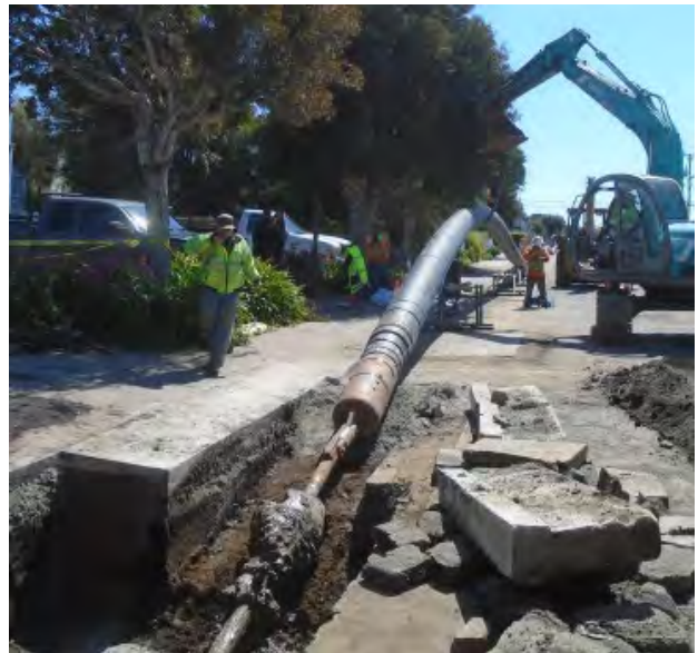
Figure 3 – Example of pre-fabricated product pipe string [Left]; Pullback of product pipe [Right]
