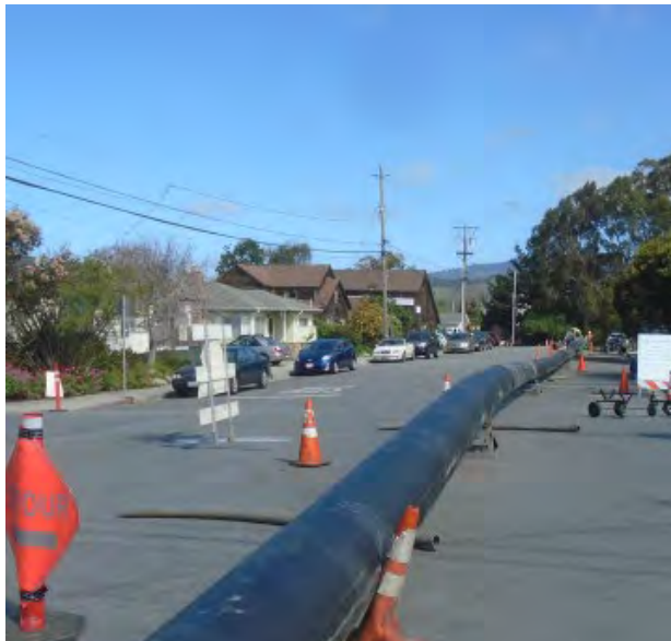
Figure 3 – Example of pre-fabricated product pipe string [Left]; Pullback of product pipe [Right]
