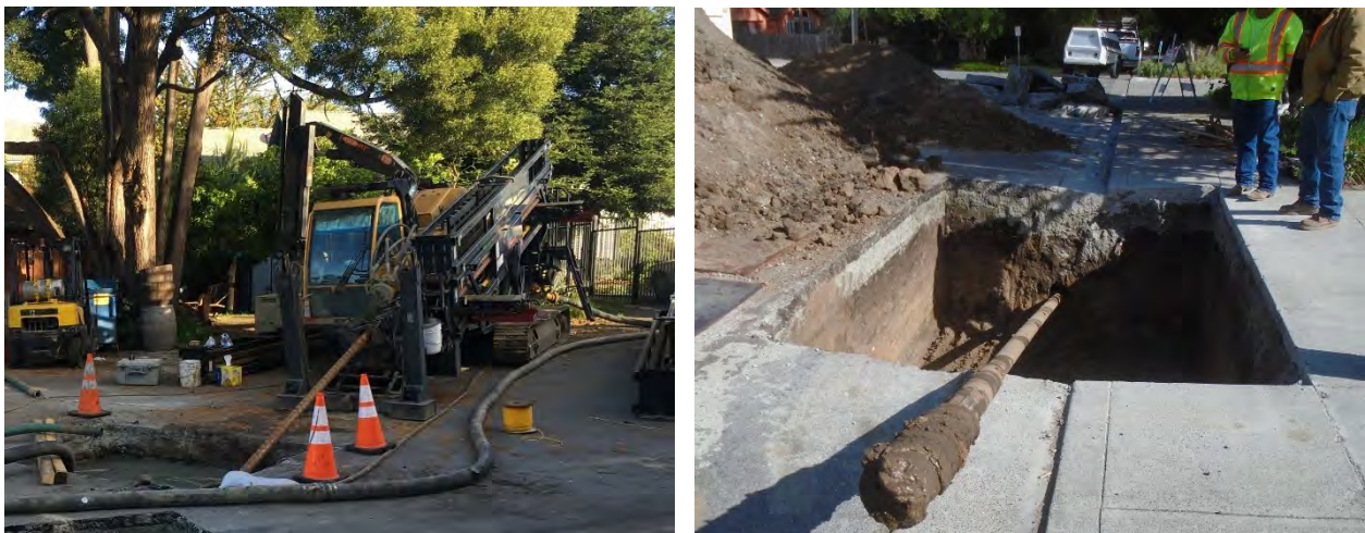
Figure 2 – HDD drill rig installing pilot bore [Left]; Pilot bore drill bit at exit pit [Right]
