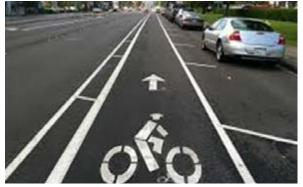
Class II: Bicycle Lane with a travel lane buffer and a parking lane buffer -Source: Kimley-Horn
