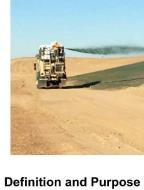
Hydroseeding typically consists of applying a mixture of wood, fiber, seed, fertilizer, and stabilizing emulsion with hydromulch equipment, which temporarily protects exposed soils from erosion by water and wind.
