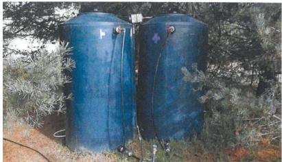
Figure 4- Two 500-gallon Mixing Tanks. (photo from 1600 Addendum)
