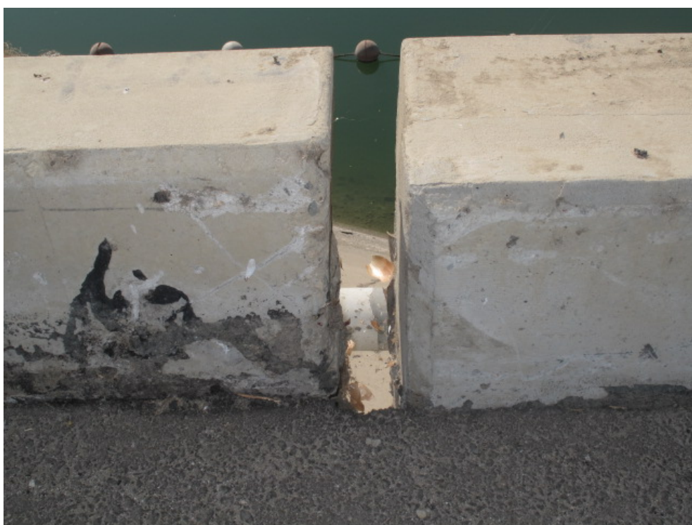
Horizontal displacement of the rail at an abutment can be seen in this image.
