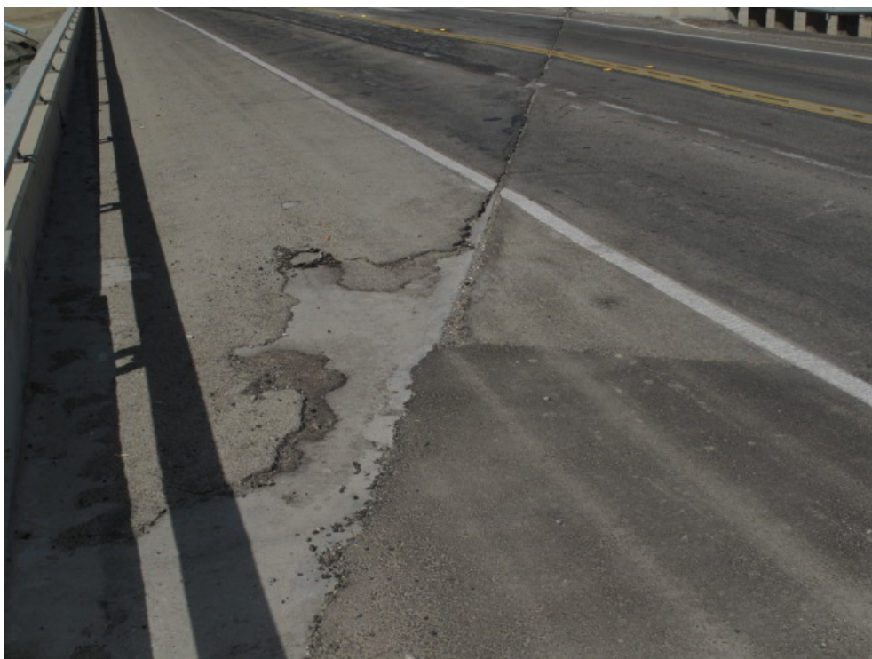
Asphalt concrete cracking at an abutment can be seen in this image.
