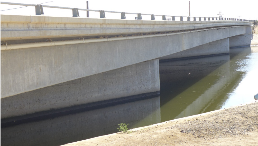
The bridge deck is sagging and is no longer visibly level in this image.
