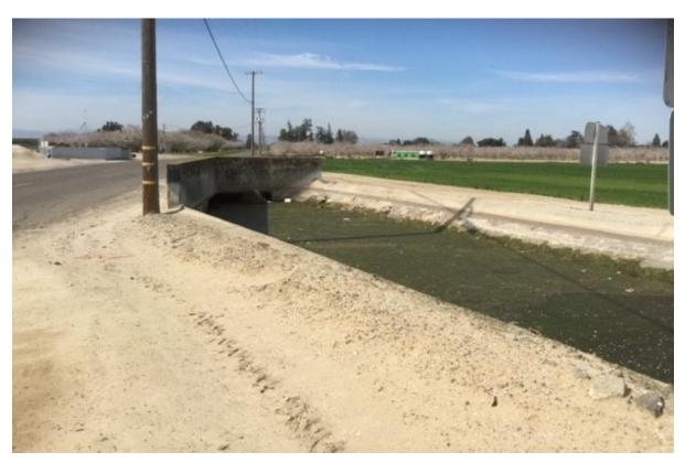
Photo 5. Concrete lined irrigation canal (Lateral #6)
