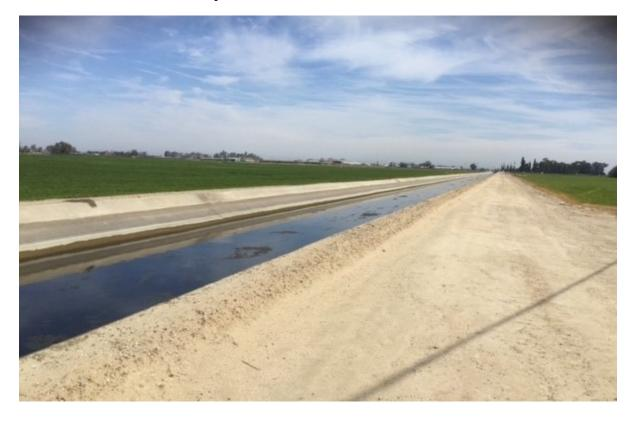
Photo 4. Concrete lined irrigation canal (Lateral #6)
