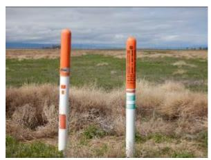
Photo #13 Typical view of fiber optic cable markers located along the eastern boundary of the site.
