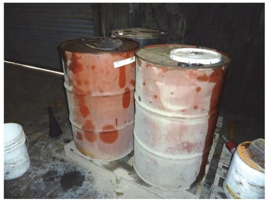
E-11. Drums of waste oil without secondary containment in mechanical shop with stains and oil sorb prominent (11/19/2019).
