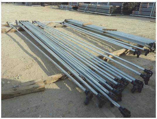
E-26. Loose drive shaft for solar power arrays in Rig Runner area with stacks of same in background (11/19/2019).
