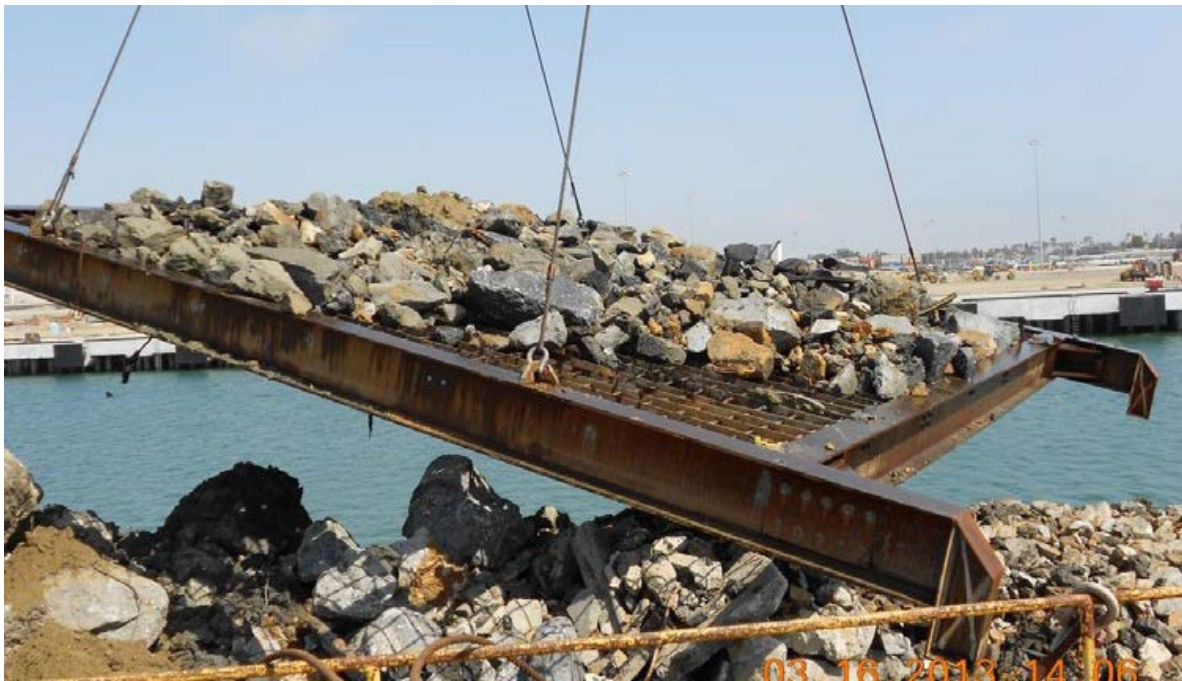
Figure 6 Examples a) Large scow with movable steel grizzly in the Port of Oakland (CA). b) Debris captured on 1-ft square grizzlies (California). Photos from DMMP 2015.
