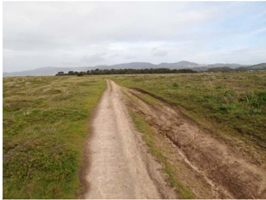
Photo 12: Photo of erosion caused by runoff collected along Beach Avenue and draining toward Gully 8. The project proposes to rehabilitate this segment of road by ripping the road tread and reseeding. Small dips will also be installed to disperse runoff.
