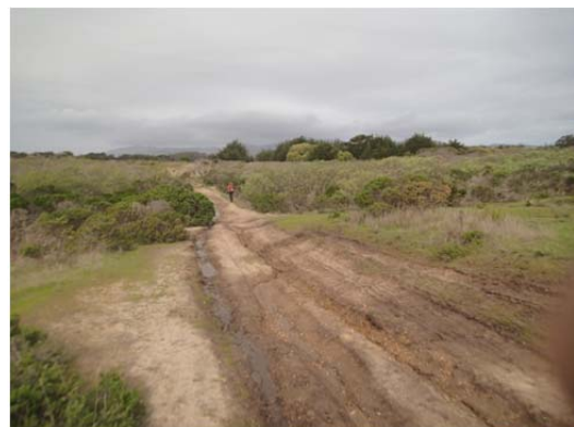
Photo 14: Erosion of Park Avenue on the south side of Ravine 9 due to poor road drainage. This photo was taken before the large dips were installed at the base of the road. For long term stability additional dips will need to be installed, the road surface rocked and a rocked road ditch constructed.
