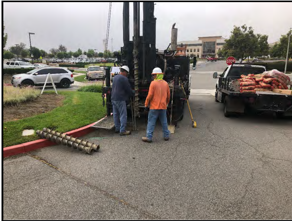
Figure 3-2. Drilling Geotechnical Test Boring B-1
