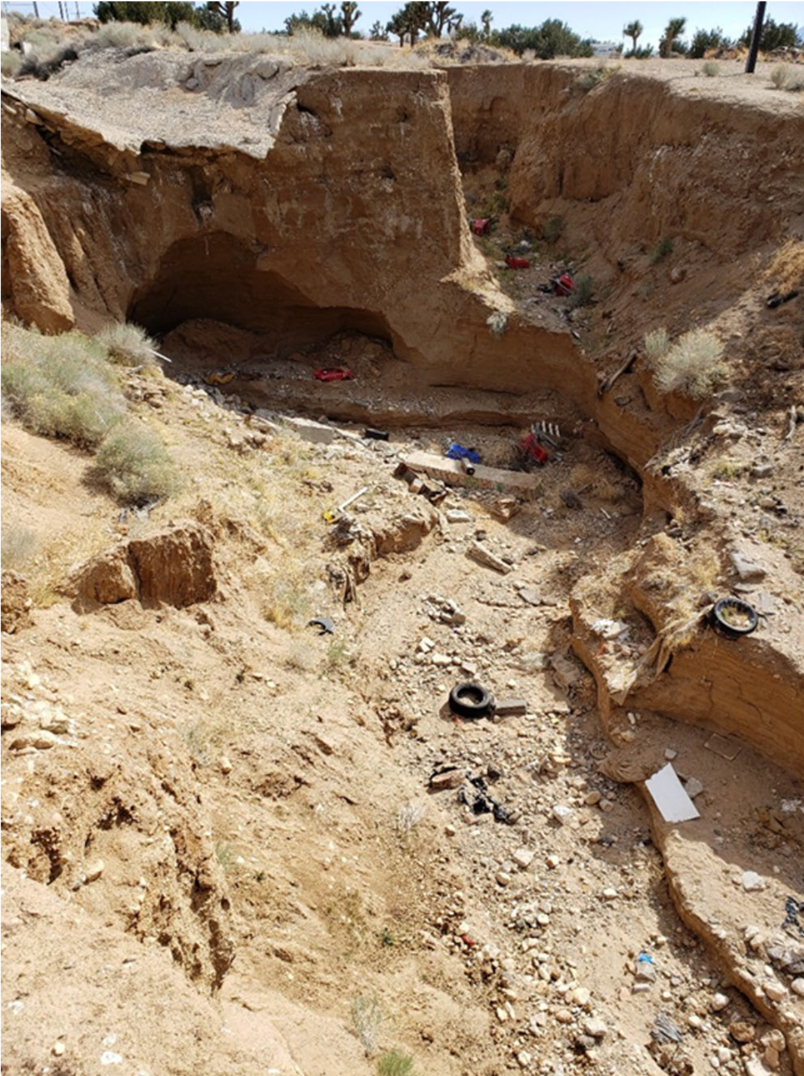
Attachment 1. Erosion immediately downslope of Cataba Road storm drain concrete discharge apron.
