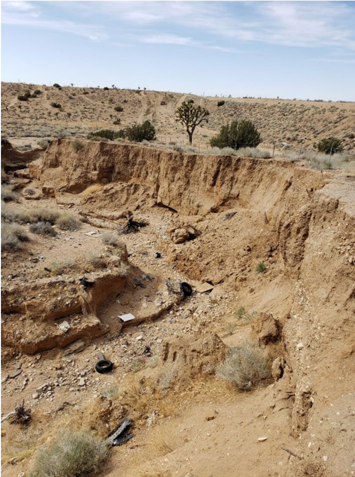
Attachment 2. Erosion channel scoured downslope of Cataba Road storm drain with the Aqueduct embankment in the background.
