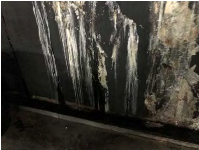
21. Tar seepage in the bottom level basement.
