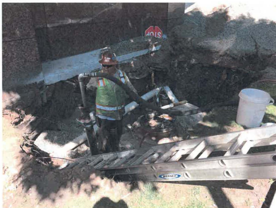
Triple Rinsing of UST with Potable Water and Collection of Rinsate Fluid via a vacuum truck
