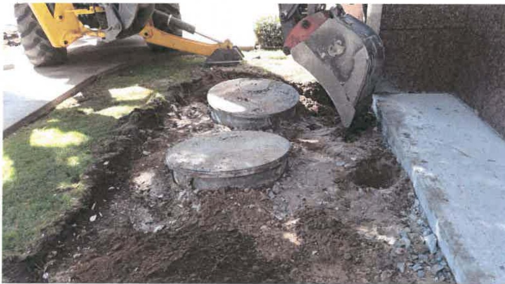
Removing top soil using an excavator
