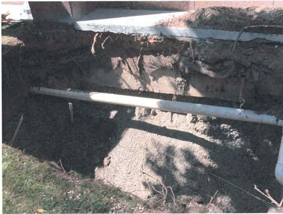
Tank Cavity left in the ground after the UST was removed
