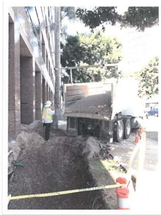
Backfilling with imported pea gravel
