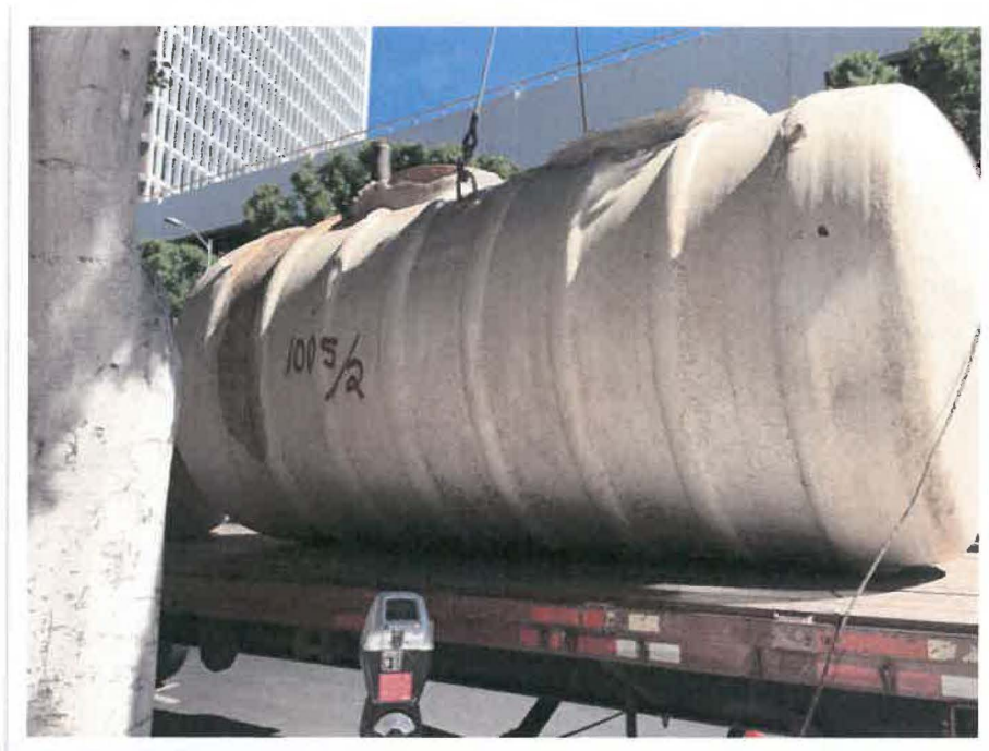
UST removed from ground and loaded onto a flatbed truck
