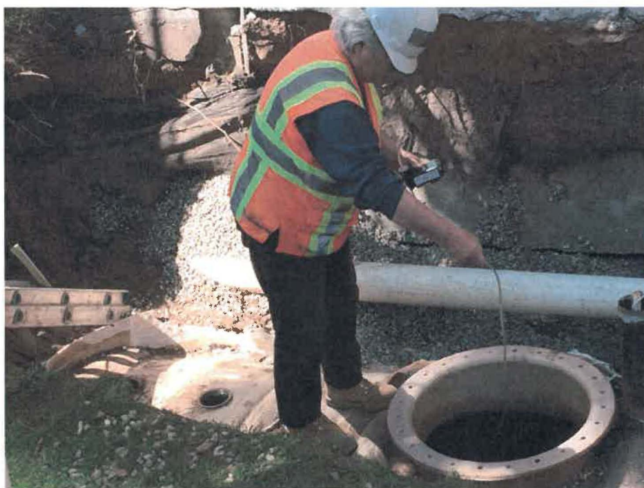
Triple Rinsing of UST with Potable Water and Collection of Rinsate Fluid via a vacuum truck
