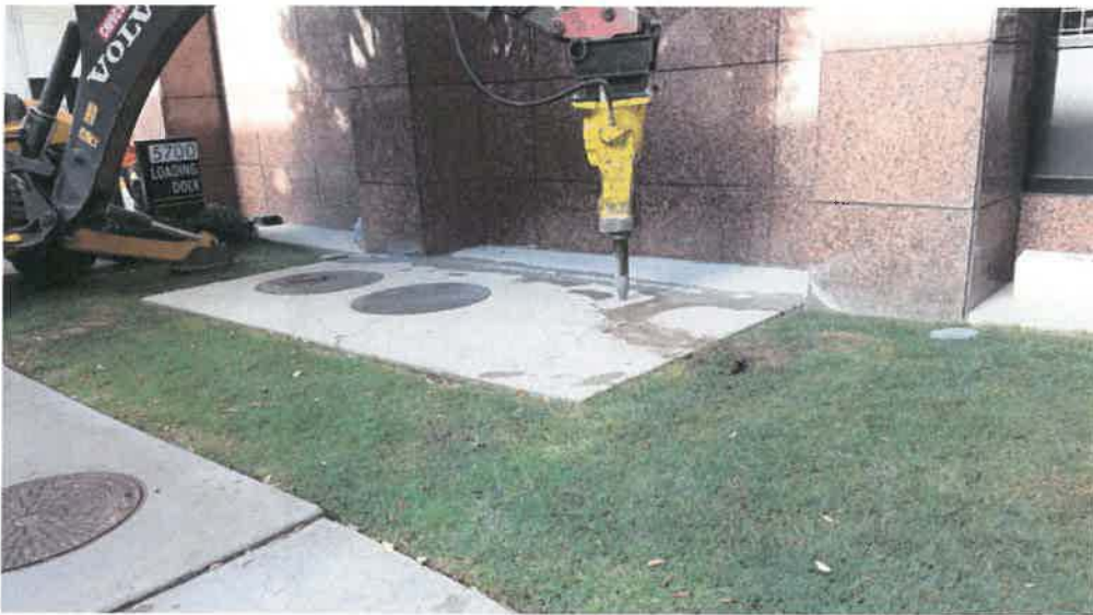
Breaking Concrete with hydraulic hammer attachment
