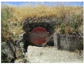
Photo 17. The flapgate on the northernmost culvert outlet on the Outfall Channel. This arm of the channel was dry during fieldwork in February and June. 17 June 2020.
