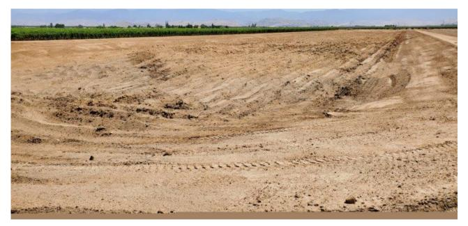
Photos 3 (above) and 4 (below): Western phase 1 basin. This basin was newly constructed and entirely barren of vegetation at the time of the August 4 field survey, save the northwestern corner (below) where an existing agricultural basin had been merged into the new basin.
