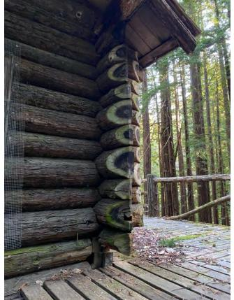
Figure 4. Close up of the cabin's typical saddle notching, facing northeast.
