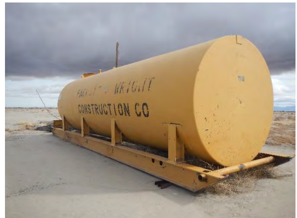
Photo #46 View of the ~20,000-gallon red dye diesel AST located on the northern portion of Tract 4 of the site.
