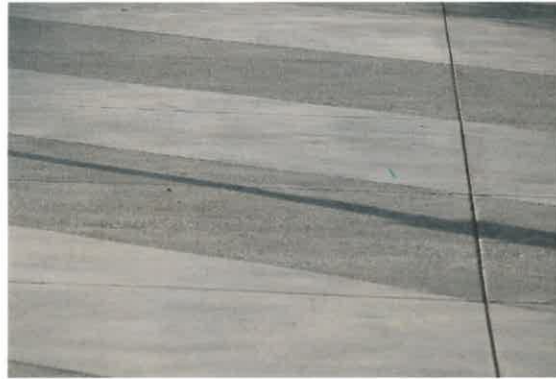
CONCRETE PAVING WITH ALTERNATING FINISH FINISH TO BE LIGHT BROOM AND ACID ETCHED
