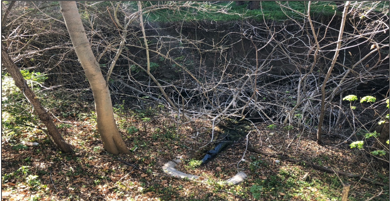
Photograph 3. Photograph was of the existing 4-inch discharge pipe that discharges stormwater from the station into Agua Fria Creek. Photograph was taken on February 11, 2020.
