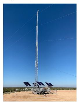
Sample Mid-Deployment Telescoping Lattice Tower Set on Center Support Pole
