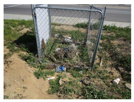
**Photograph 11:** Riser on the northeast corner of the project site that connects into the adjacent underground stormwater system along Perris Boulevard.
