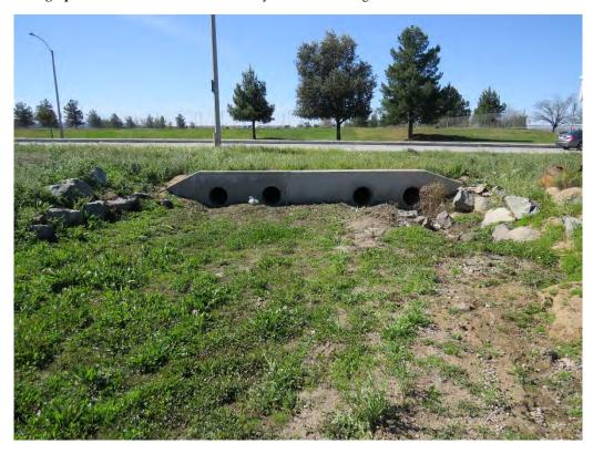
**Photograph 20:** Looking at the western terminus of the swale where it extends under Indian Avenue, via four 24-inch culverts, and connects with a water detention basin on the southwest corner of the intersection of Ramona Expressway and Indian Avenue.
