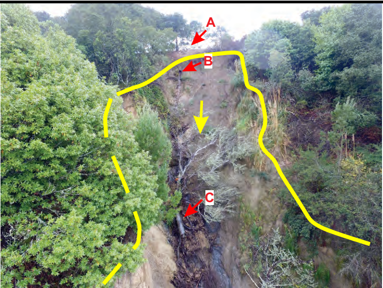
Image 1. South view of 12/04/19 erosional gorge & escarpment from storm drain pipe. A is edge of roadway; B is current CMP outfall; C is detached pipe segment.
