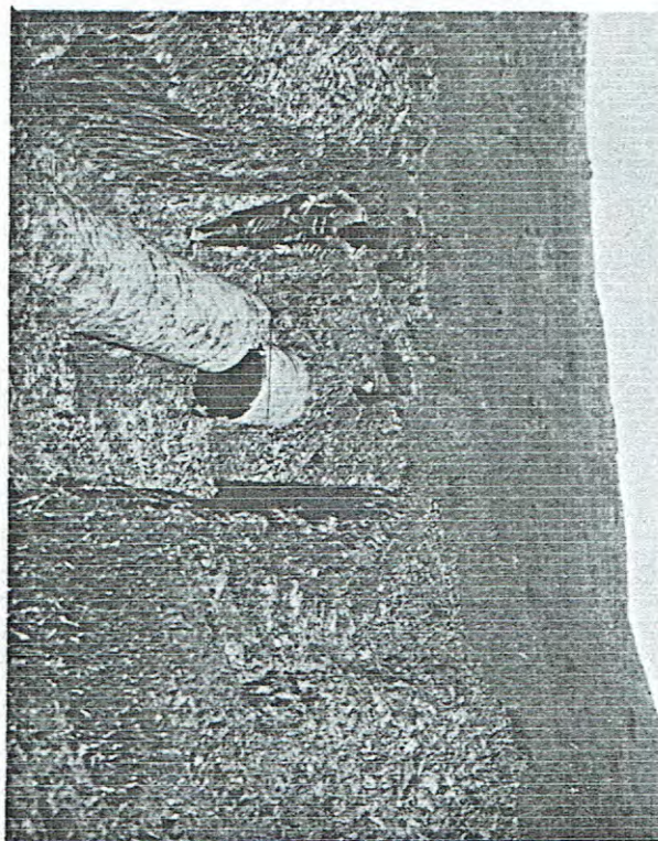
A. Offset in 30-inch water-pipe by fault, Northwest of San Andreas Lake, A. O. L.
