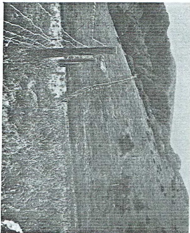
B. Collapse of 30-inch water-pipe northwest of San Andreas Lake, R. L. H.
