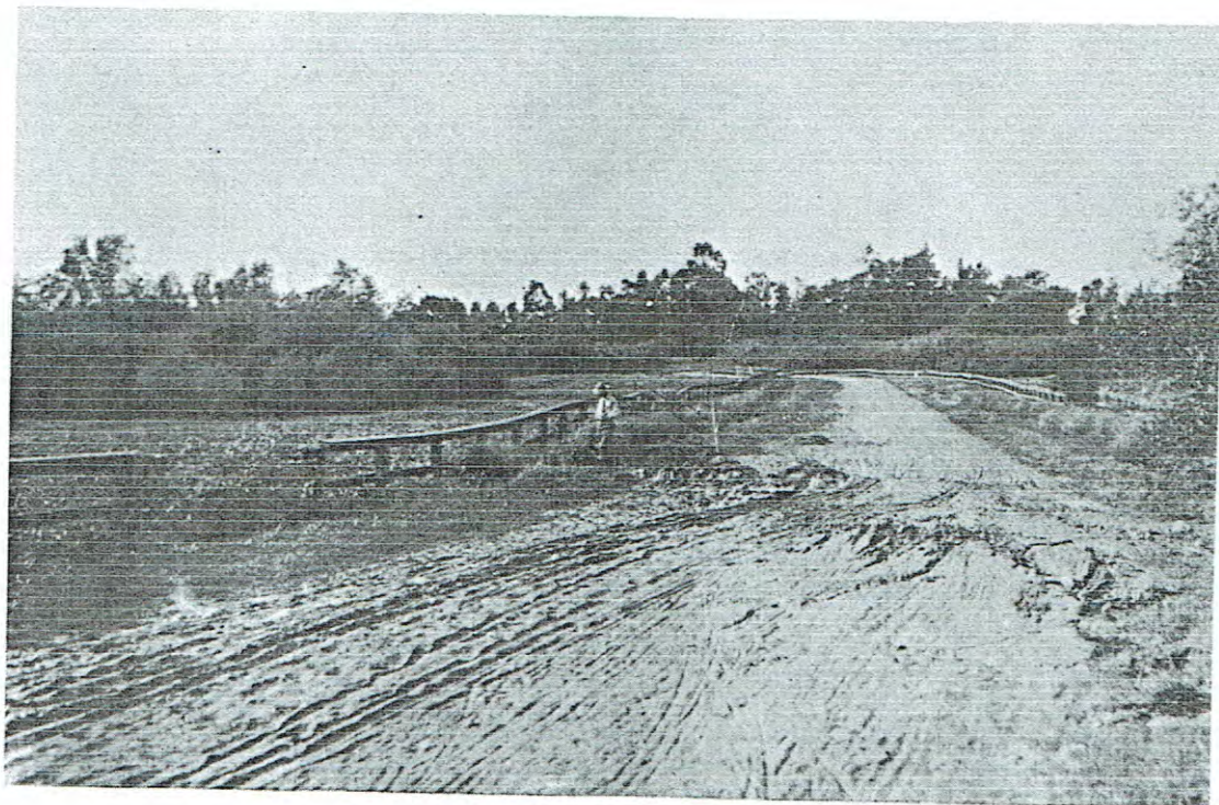
B. Offset of road by main fault near Searsville reservoir. Per J. C. B.
