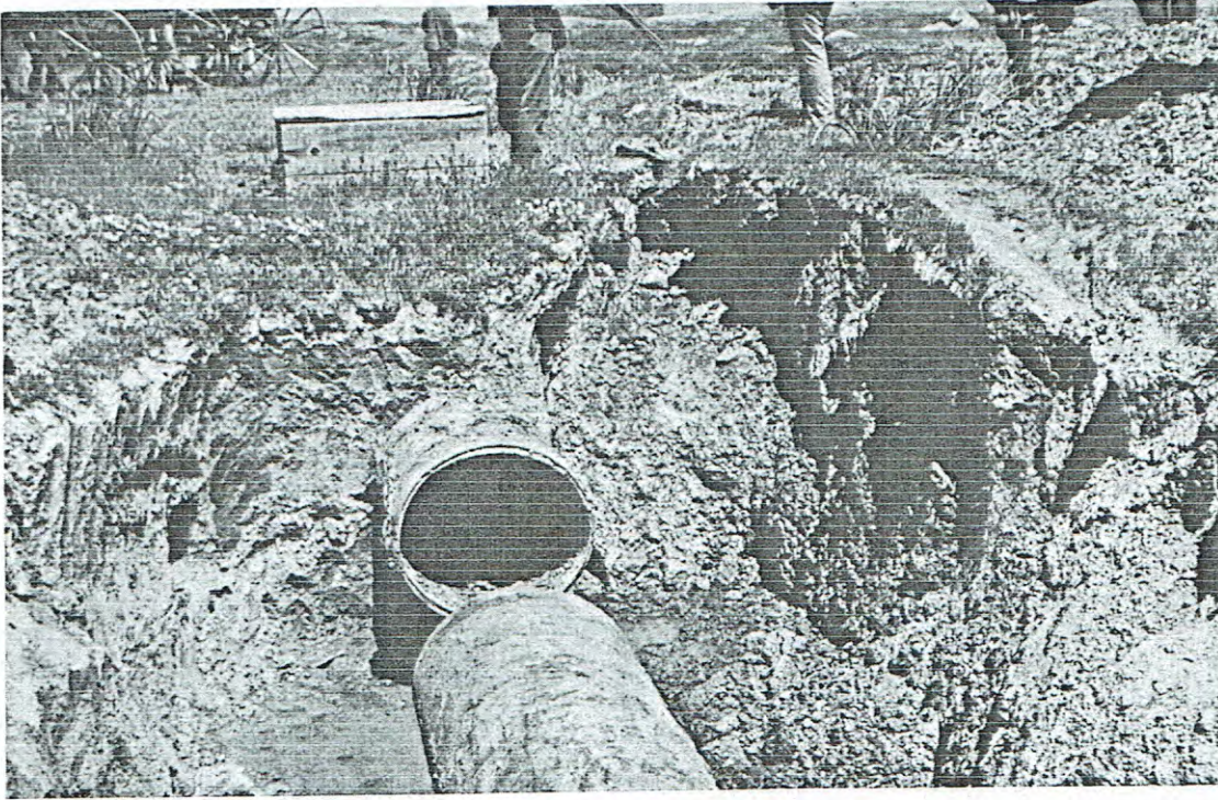
A. Rupture of 30-inch water-pipe by fault. Northwest of San Andreas Lake. A. C. L.
