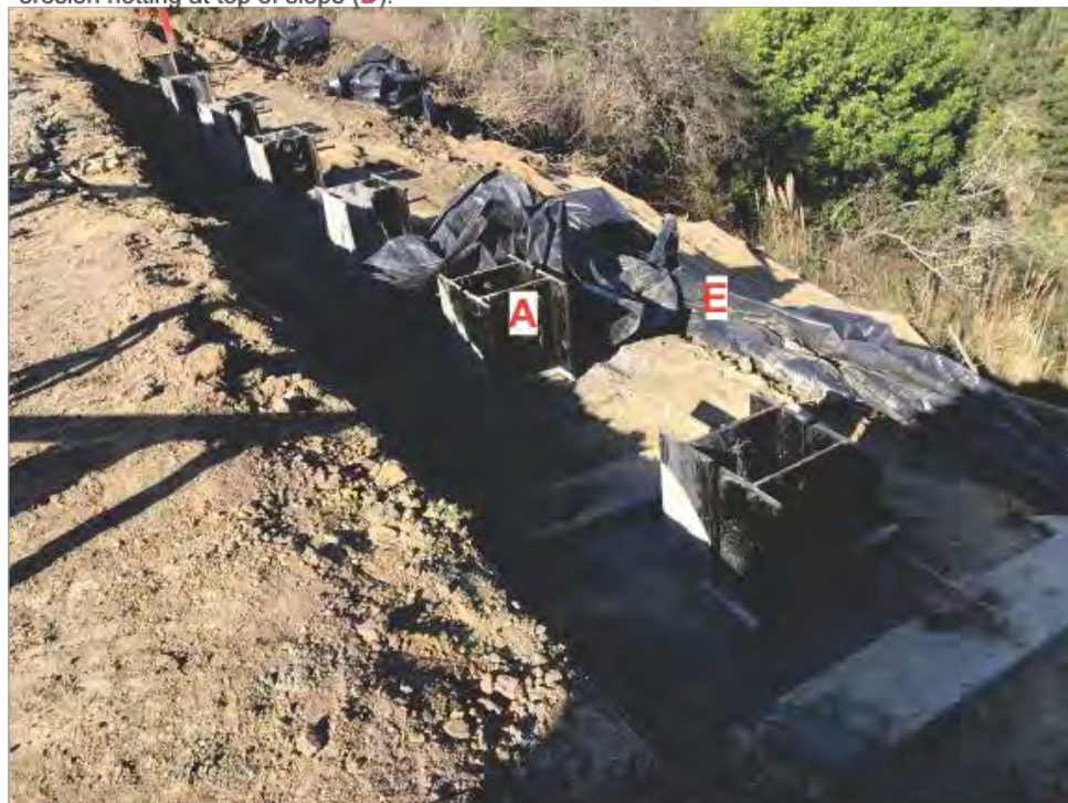
Photo 2. Westerly view along top of slope line of double I-beam reinforced concrete stitch piers (A). Edge of west-bound lane of San Bruno Avenue on left of view. Temporary plastic tarp (E).
