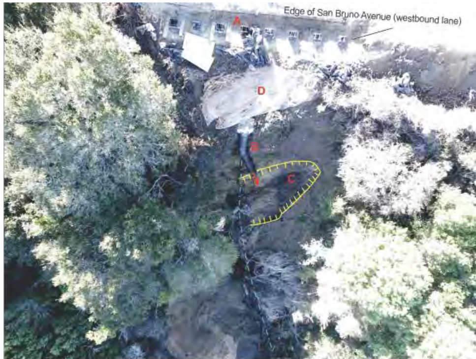
Photo 1. Aerial image of storm drain outfall, including stitch piers (A), and new HDPE outfall pipe (B), at least 20 feet above the established drainage course (blue dot-dash line). Yellow hachured line denotes gully erosion from runoff since pipe was installed (C). Temporary erosion netting at top of slope (D).
