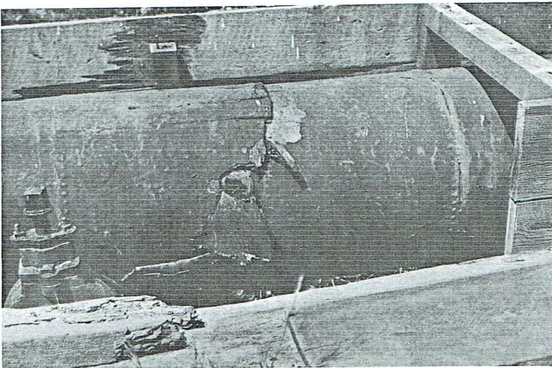
B. Thrust of 30-inch water-pipe by fault, northwest of San Andreas Lake. Amount of telescoping is 58 inches. A. C. L.
