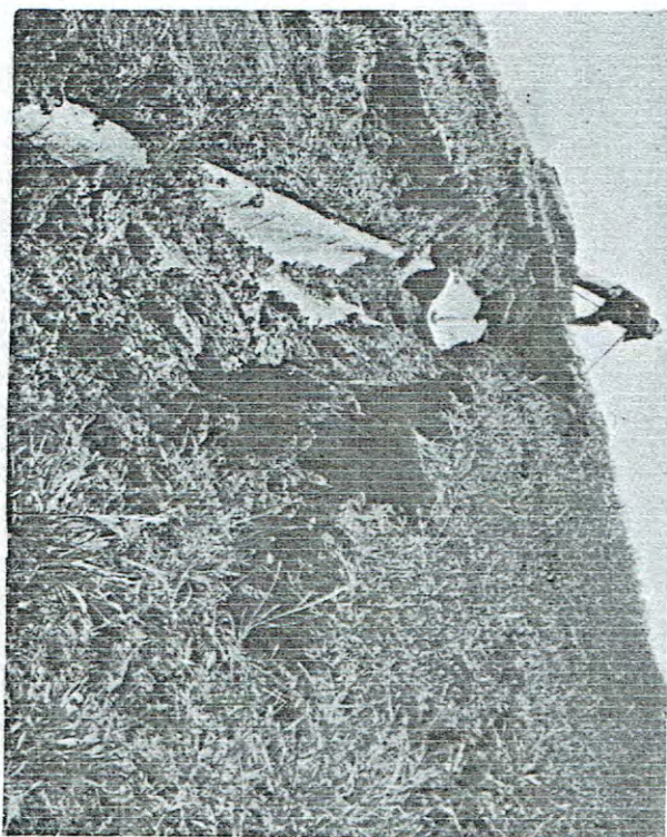
B. Collapse of 30-inch water-pipe northwest of San Andreas Lake, R. L. H.
