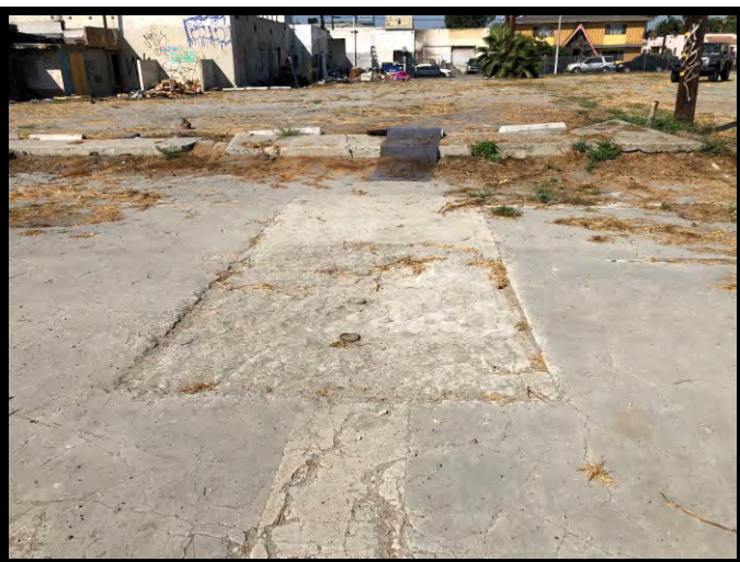
Photo #5: View of concrete cutout in area of former gas station structure.
