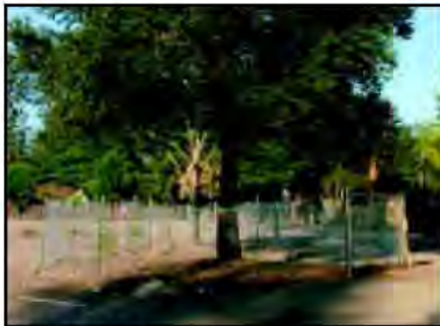
IMAGE 2.15-2 Tree Protection Fence at the Dripline
