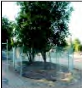
IMAGE 2.15-1 Tree Protection Fence at the Dripline
