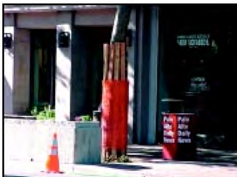
IMAGE 2.15-4 Trunk Wrap Protection
