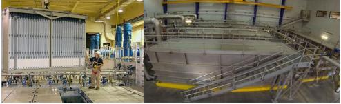
Image 2-11a MBR Filtration Module at the WWTP
