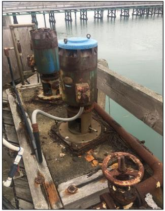
Image 2-14 RMT II-Existing Water Intake Pumps
