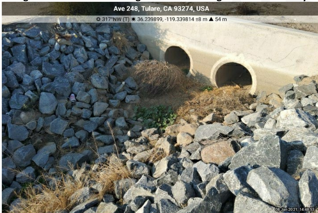
Figures 23 – Culvert of Irrigation Ditch Along Eastern Boundary
