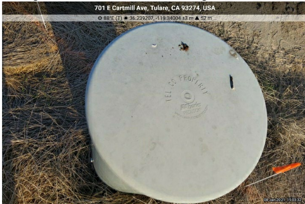
Figure 28 – Box Associated with Underground AT&T Line
