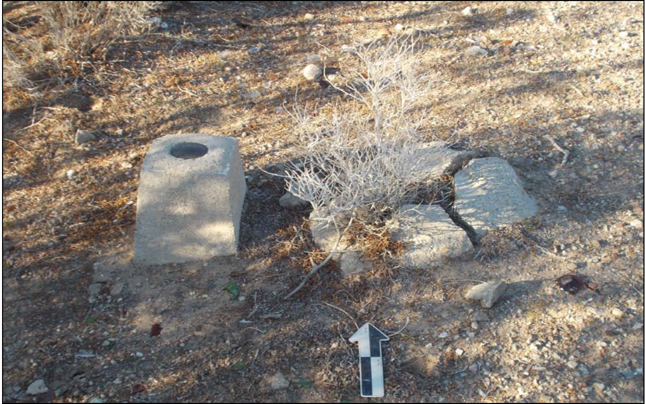
Figure 4 Overview of 1943 survey marker and older, broken survey marker that it replaced.
