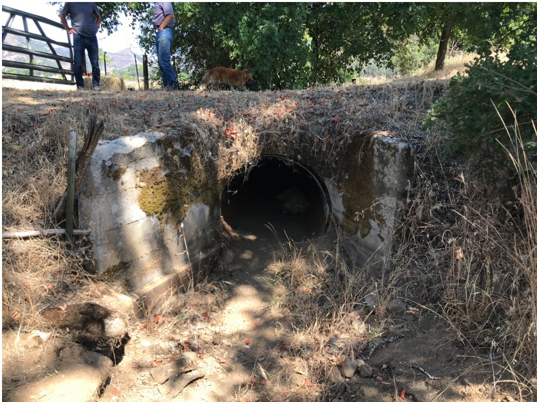
Culverted Watercourse Crossing of Project Parcel (48" CMP Culvert)
