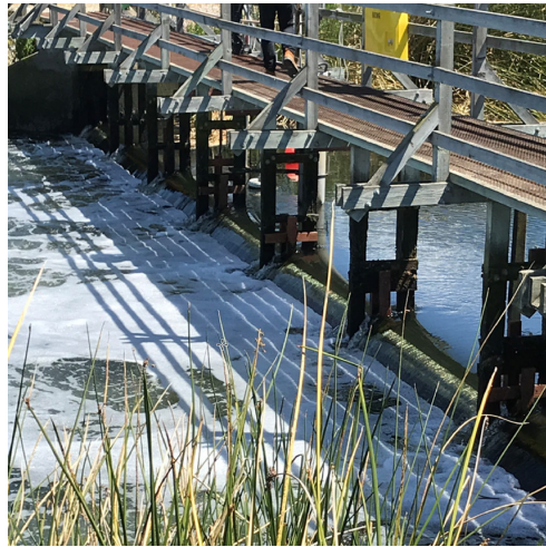
Photo 1: Existing Outfall Bridge and Weir
