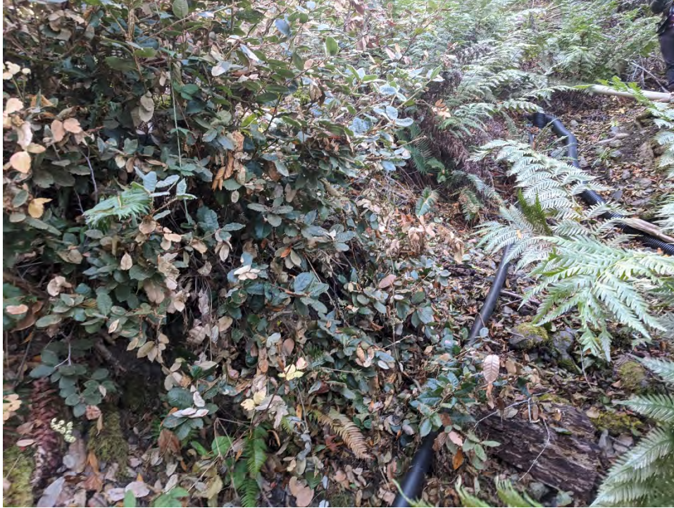
Photo 13: Water is transported to Phillipsville CSD residents via existing HDPE pipes installed above ground. Photo taken November 11, 2020.
