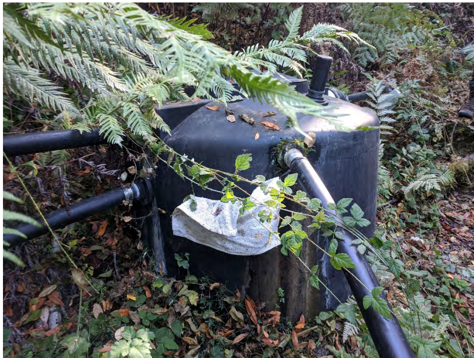
Photo 3: View of the overflow tank as part of the spring source collection system. Photo taken November 11, 2020.
