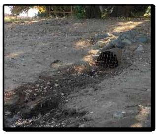
Figure 8–17. Localized stormdrain outfall with evoded outlet (~RM 0.2)
