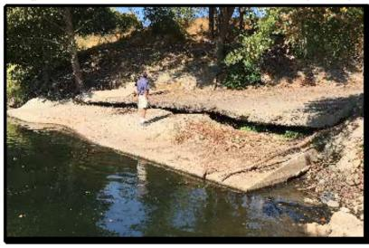
Figure 8-18. Large when stormwater cutfal with broken apron (~RM 5.3)
