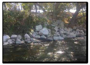
Figure 8-22. Rock rip-rap placed at Contova Creek outfall (~RM 14.5)
