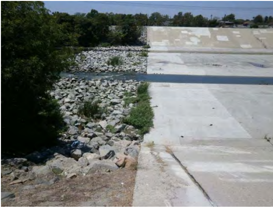
Photo 17: Upper limit of Reach 115 of the San Gabriel River from the east bank looking at the transition zone where the channel converts from concrete-lined upstream to soft bottom downstream.
