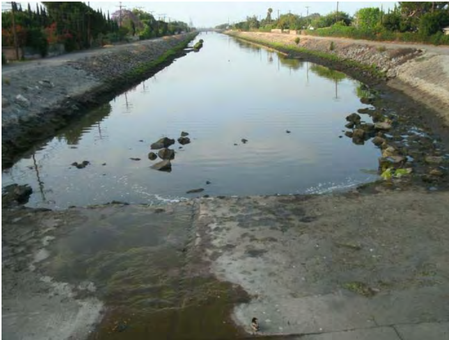
Photo 20: Los Cerritos Channel (Reach 116) facing downstream from Atherton Street bridge where the channel converts from concrete-lined upstream to soft bottom downstream.
