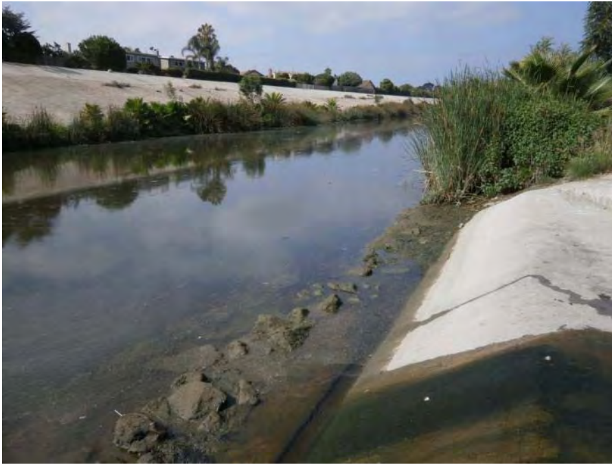
Photo 1: Ballona Creek (Reach 112) facing downstream from the northwest bank immediately downstream of Centinela Avenue. Riprap is present at the bottom of the concrete slopes.
