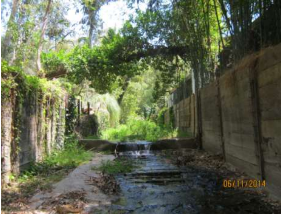
Photo 5. Southern end of the Project site. Wide section of the channel, lined with concrete. Photo showing a fallen tree across the channel. Photo facing north.
