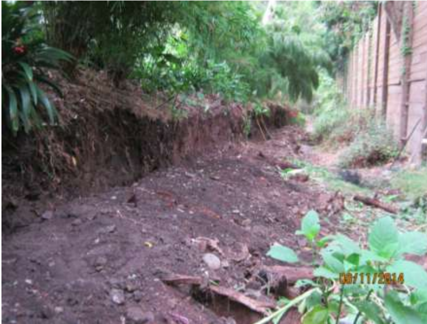
Photo 1. Photo showing removed wooden side wall on the east side of the channel, causing loose sediment to enter the channel. Photo facing south.
