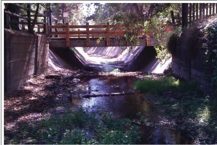
September 25, 2014. View of Reach 119, facing downstream from soil test pit 8, showing transition to concrete lined channel.
