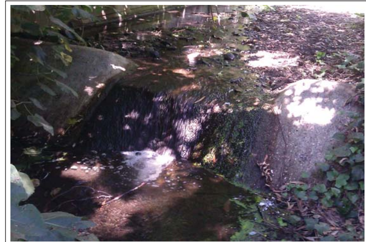
September 25, 2014. View of typical drop structure within Reach 119.
