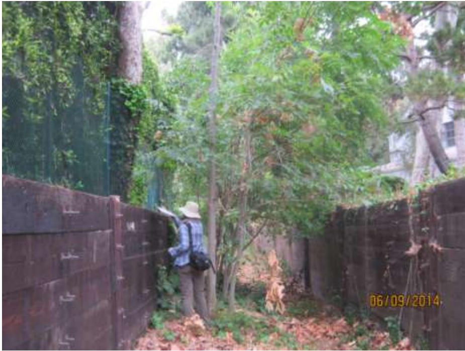
Photo 3. Section of the channel located by Rustic Creek Lane. Thick litter layer present on top of concrete lined channel. A small stand of native alders are present in the photo. Photo facing northwest.
