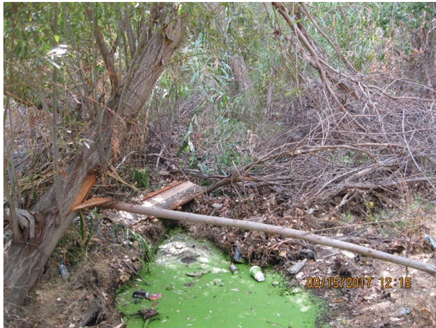
September 15, 2017 - Entrainment channel is blocked by accumulated debris at 90-degree bend.
