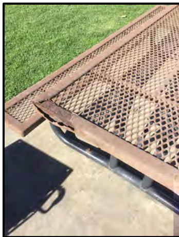
Figure 15b. Picnic Table with exposed metal
