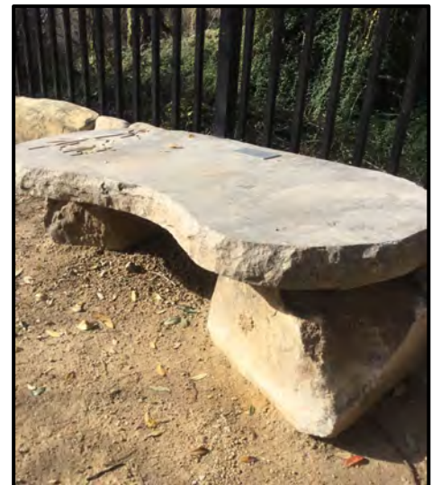
Figure 8a. Bench surface not properly secured to legs (rated 1)
